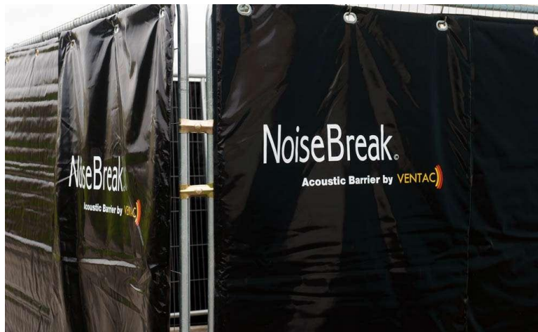
Figure 5: Temporary Construction Noise Barrier © Ventac
